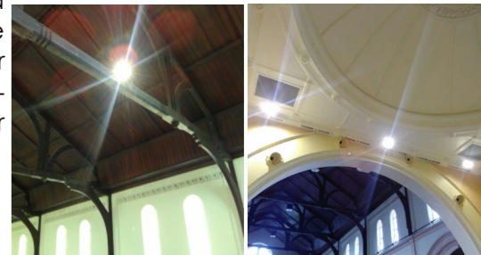
New lights installed at St Marys
